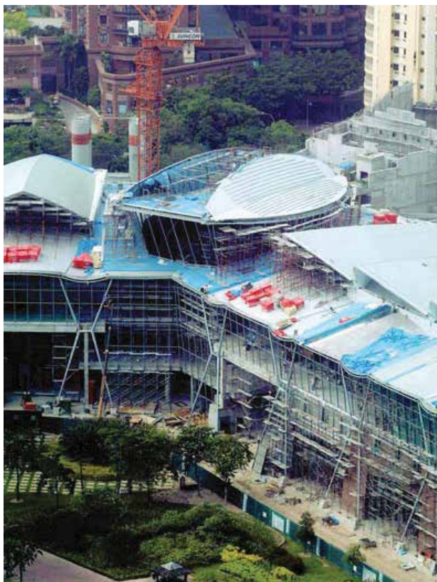
Roof installation of Kuala Lumpur Convention Centre
