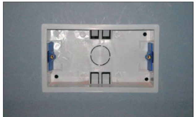
Switch box before installation of Putty Pad.
