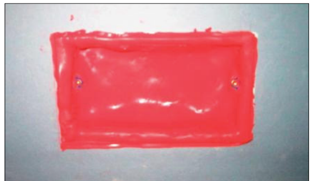
Putty Pad installed inside switch box.
